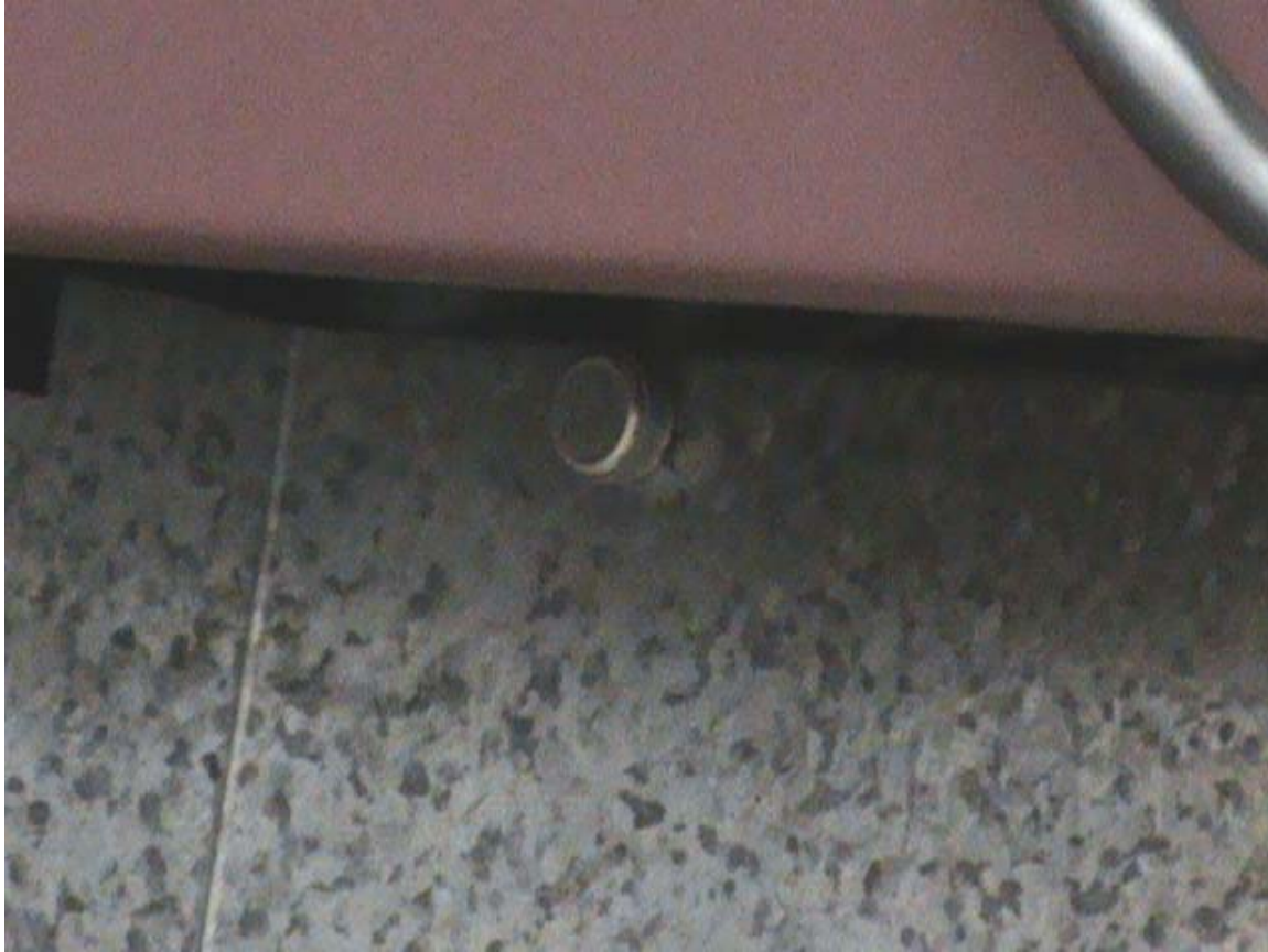
Figure 1: Security Screw - installed, with security cap which deters removal and prevents undetected removal
